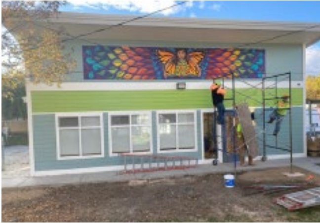
La Escuelita under construction and ready for solar.
